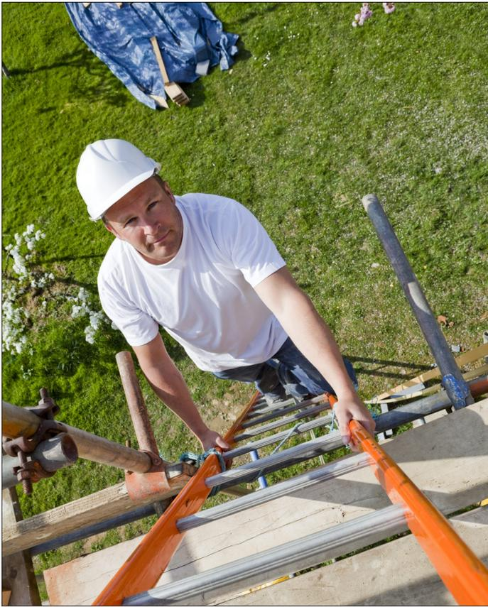
Avoid tripping hazards by keeping the area around the tip and base of the ladder clear. Do not run hoses or extension cords along the ladder's rungs where they will create a tripping hazard.
